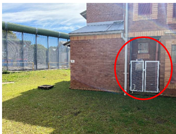
A gas hot water system attached to the wall of one of the cells in the southwest corner of the site
